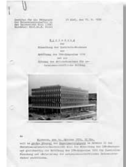
The IPN building, Olshausenstraße 62, was opened in October 1970 after a three year period of construction. The Volkswagen Foundation financed the construction.
